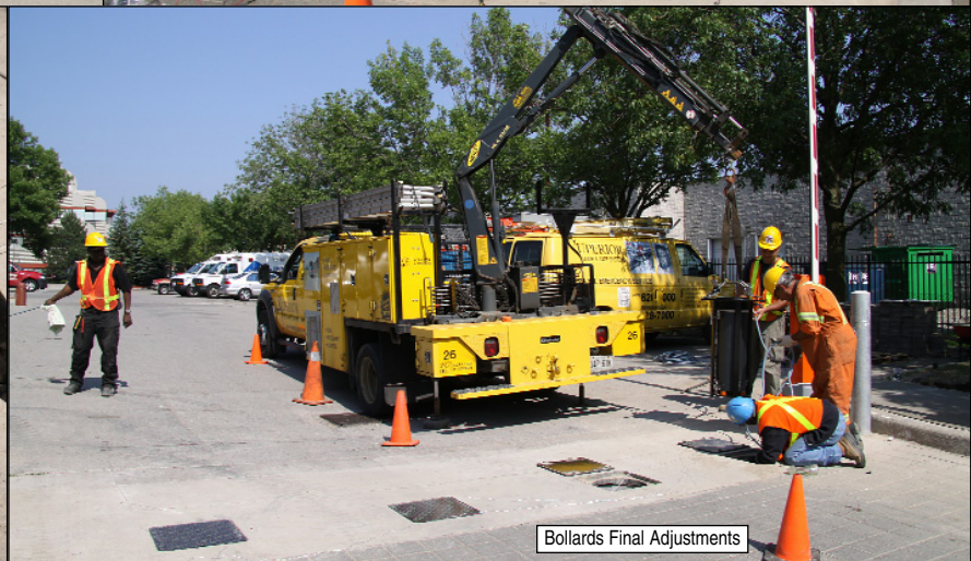
Lowering Bollards Into Enclosures
