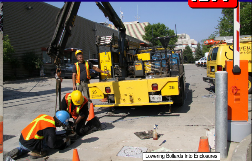
Lowering Bollards Into Enclosures
